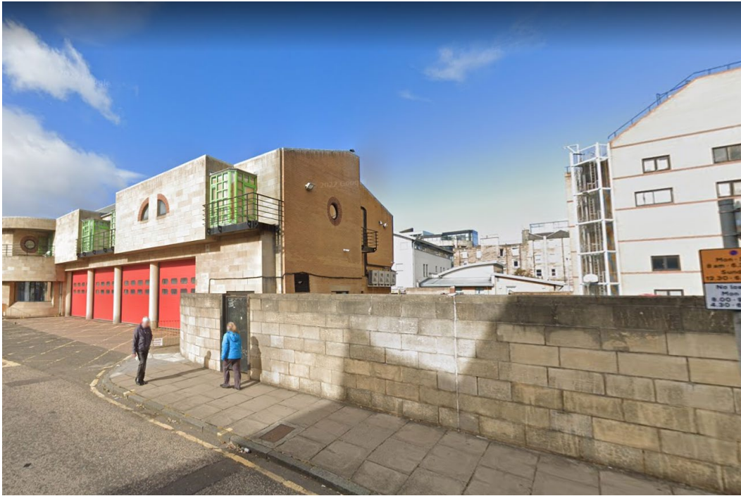
Fire station and carpark to north of site.
